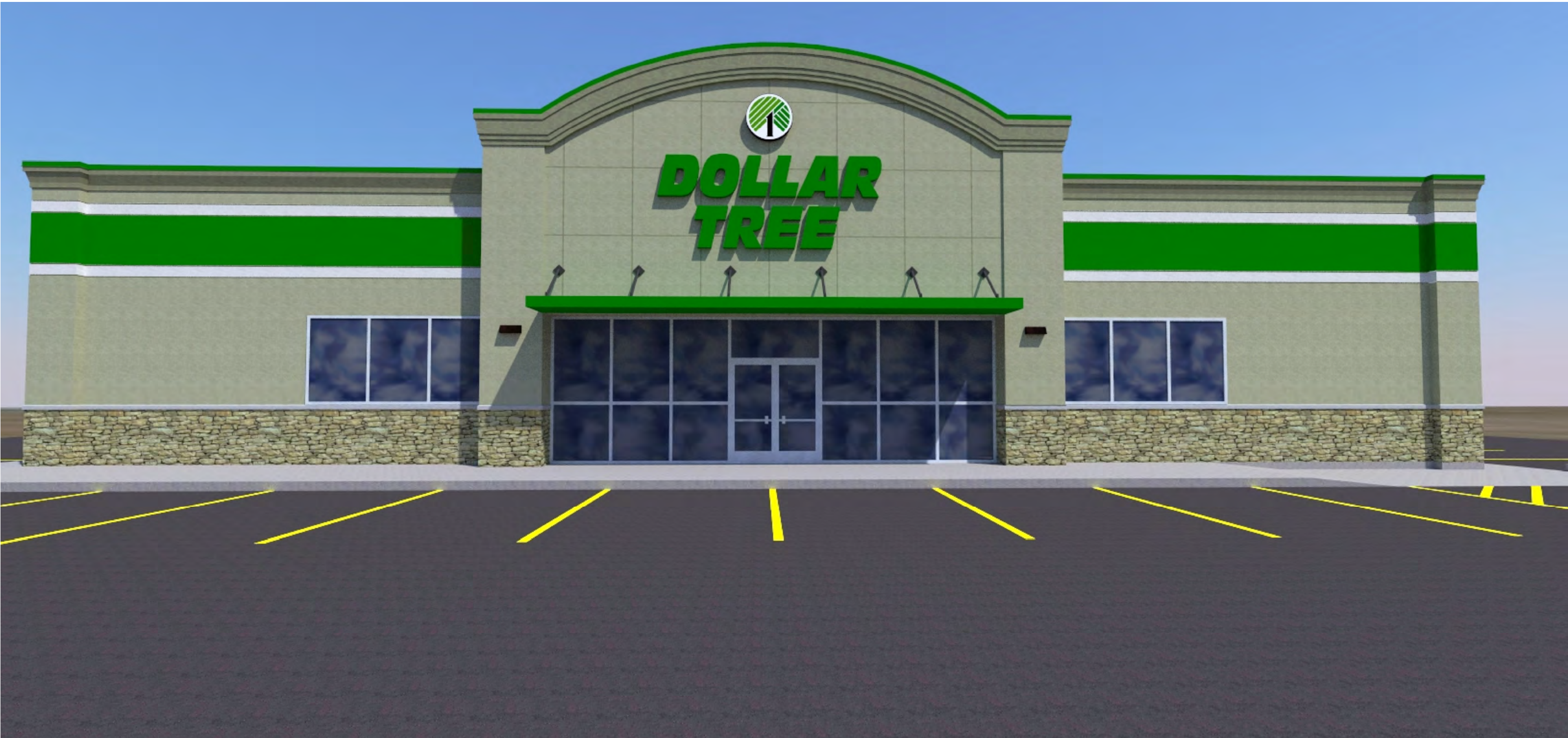
VIEW FACING TOWARD MIDDLE ROAD
